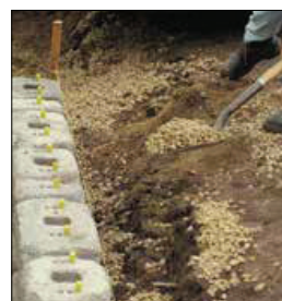
4. INSTALL FILL & COMPACTION
