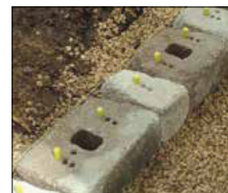
3. INSERT FIBERGLASS PINS
